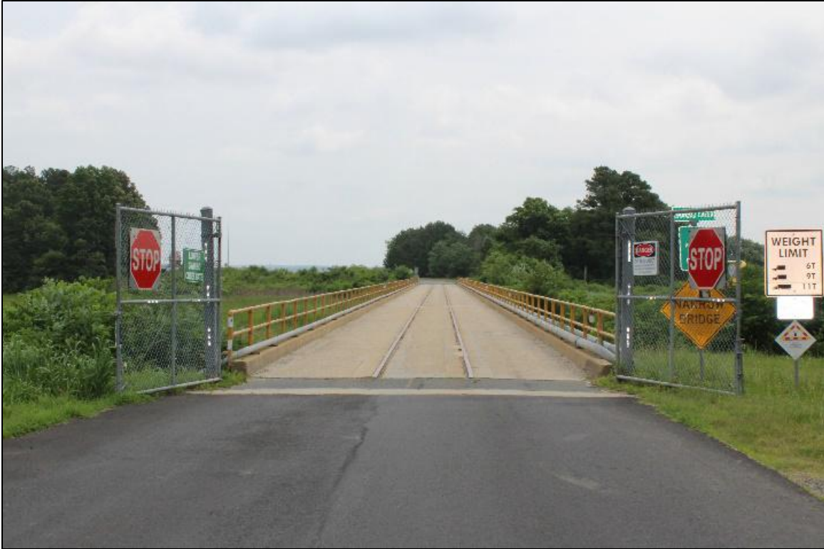
Figure 3-10 View of Gambo Creek Bridge Looking East
