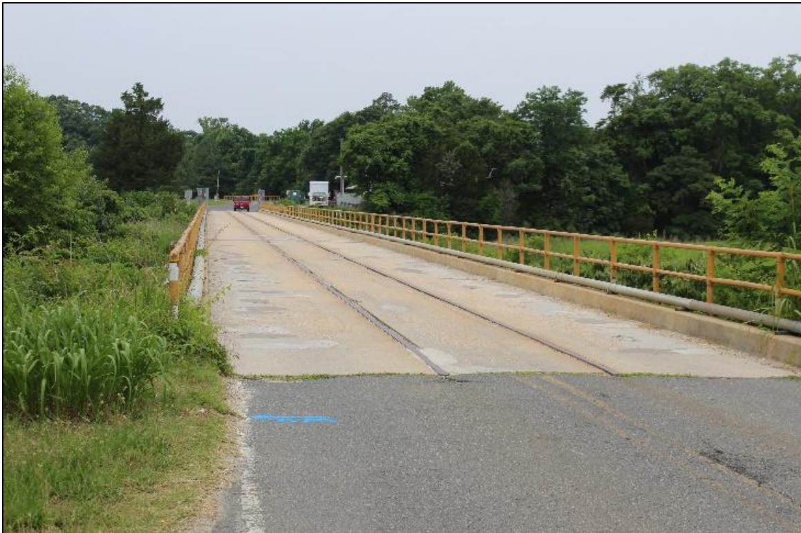
Figure 3-11 View of Gambo Creek Bridge Looking West
