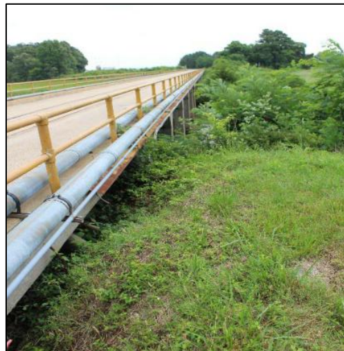
Figure 3-1 Photo of Gambo Creek Bridge Looking Northeast
